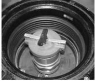
Step 2: Remove the A0099-002, -003 vapor adapter cap.
