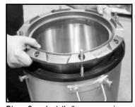
Step 8: Install the new primary insert into the existing spill containment. Use the studs to assist with alignment.
