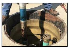
Step 2: Remove the Model A1100 OPV from the tank fill riser.
