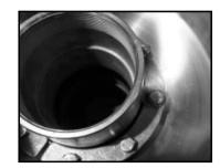
**Step 12:** Use the eighth 9/16" flange bolt and washer to install the new grounding clip. Be sure the grounding clip touches the female coupling.
