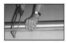
4. Carefully cut the top drop tube to the required length. Use a hacksaw equipped with a fine tooth blade to ensure a straight 90-degree cut.
