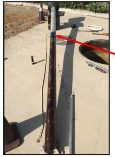
Step 3: Place the Model A1100 OPV on its side with the primary float facing downward. *Refer to Figures 1 and 2 for details.*
