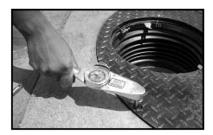
Fasten the manhole lid to the manhole rim. Manually install the factory supplied 5/16 Allen hex bolts to avoid cross threading. Tighten and torque between 9 and 11 ft-lbs.
