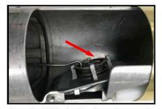
**Step 8:** With the hook end secured, gently allow the flapper valve to move upward and spring back into an open position, tug gently on the test tool, the flapper valve must relatch and remain open.
