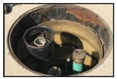
Step 1: Remove the spill container lid, fill cap and adapter from the tank fill riser. Note: only remove manhole cover and water shroud system if necessary.
