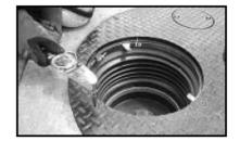
4. Fasten the A1004EVR spill containment fill and vapor to the bottom of the manhole. Manually install the factory supplied 5/16 Allen hex bolts to avoid cross threading. Tighten and forque between 9 ft and 11 ft-lbs.
