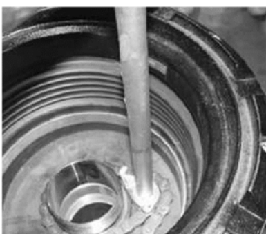
Step 5: Use a standard 1/2" drive ratchet and chain wrench to loosen and remove the containment nipple.
