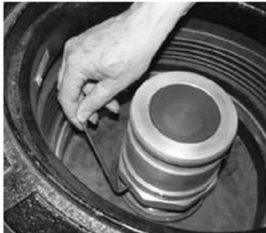
Step 3: Use a 5/32" allen wrench to loosen and remove both set screws from the base of the A0076-124S swivel vapor adapter.
