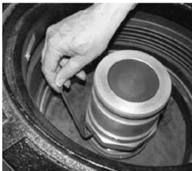
Step 3: Use a 5/32" allen wrench to loosen and remove both set screws from the base of the A0076-124S swivel vapor adapter.
