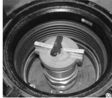
Step 2: Remove the A0099-002, -003 vapor adapter cap.
