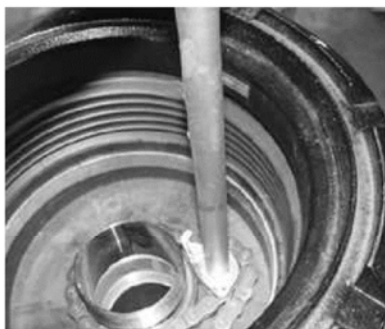
Step 5: Use a standard 1/2" drive ratchet and chain wrench to loosen and remove the containment nipple.
