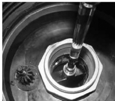
Step 6: Use the EMCO Riser Seal Wrench p/n 494120 to loosen and remove the center insert located inside the 494096 riser seal.
