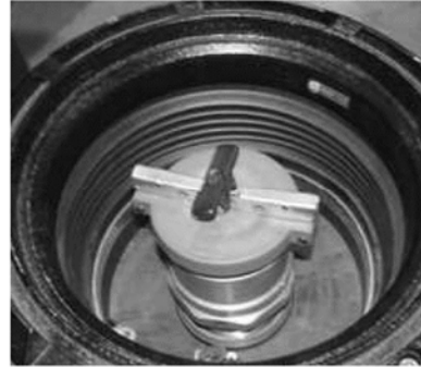
Step 2: Remove the A0099-002, -003 vapor adapter cap.
