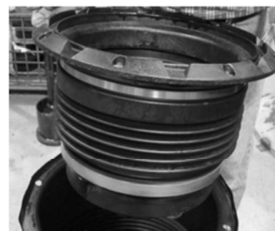
Step 12: Remove the primary liner from inside the A1004EVR spill containment by pulling upwards. Once the primary liner is completely out, please discard.
