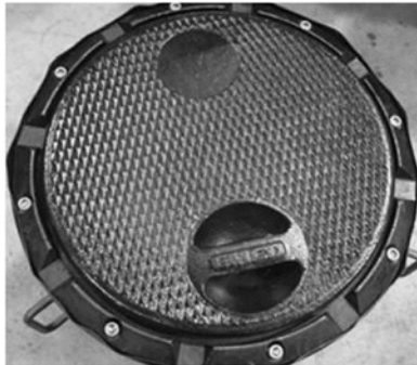
Step 1: Remove the A1004EVR spill containment lid.
