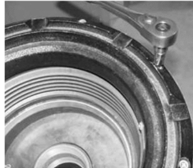
Step 6: Use a ratchet with a 3/8" socket or 1/4" allen wrench to remove and discard all eight 3/8" stainless steel bolts located along the top of the rim of the A1004EVR spill containment.
