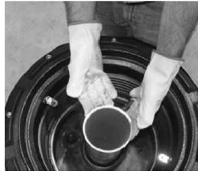
Step 8: Remove the drop tube from the fill riser by pulling upward.
