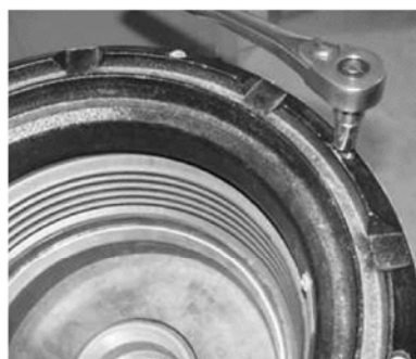
Step 6: Use a ratchet with a 9/16" socket to remove and discard all eight 3/8" stainless steel bolts located along the top of the rim of the A1004EVR spill containment.
