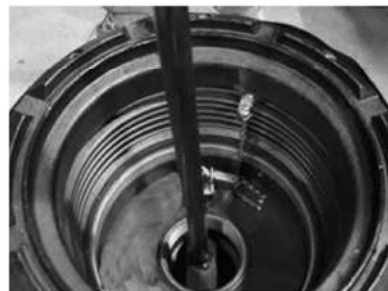
Step 10: Use the EMCO Spill Containment Wrench p/n A0081-001H to loosen and remove the primary liner from the fill riser pipe.
