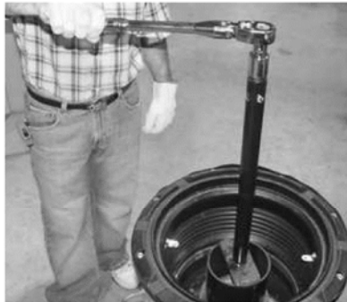
Step 7: Use the EMCO Adapter Wrench p/n A0081-001C to loosen and remove the 494096 riser seal.
