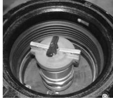
Step 2: Remove the A0099-002, -003 vapor adapter cap.
