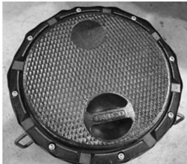
Step 1: Remove the A1004EVR spill containment lid.
