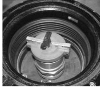
Step 2: Remove the A0099-002, -003 vapor adapter cap.
