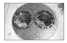
5. Fasten the A1004EVR spill containment lid rims fill and vapor to the top of the manhole lid. Manually install the factory supplied 5/16 hex bolts to avoid cross threading. Tighten and torque between 9 ft and 11 ft-lbs.
