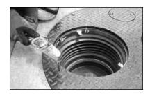
4. Fasten the A1004EVR spill containment fill and vapor to the bottom of the manhole. Manually install the factory supplied 5/16 Allen hex bolts to avoid cross threading. Tighten and torque between 9 ft and 11 ft-lbs.
