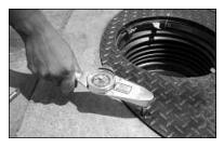
Fasten the manhole lid to the manhole rim. Manually install the factory supplied 5/16 Allen hex bolts to avoid cross threading. Tighten and torque between 9 and 11 ft-lbs.
