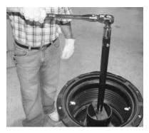
Step 7: Use the EMCO Adapter Wrench p/n A0081-001C to loosen and remove the 494096 riser seal.
