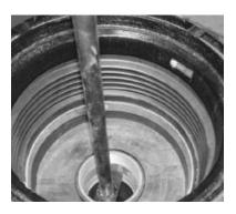
Step 7: Use the EMCO Spill Containment Wrench p/n A0081-001H to loosen and remove the primary liner from the vapor riser pipe.
