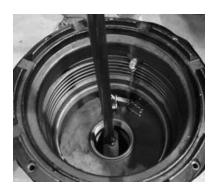
Step 3: Manually tighten the new primary liner onto the riser pipe to avoid cross threading. Use the EMCO Spill Containment Wrench p/n A0081-001H to tighten and torque between 100 and 150 ft-lbs.
