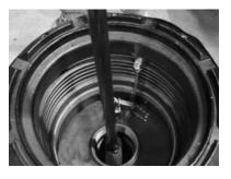
Step 10: Use the EMCO Spill Containment Wrench p/n A0081-001H to loosen and remove the primary liner from the fill riser pipe.
