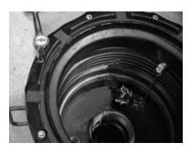
Step 9: Use a ratchet with a 3/8" socket or 1/4" allen wrench to remove and discard all eight 3/8" stainless steel bolts located along the top of the rim of the A1004EVR spill containment.
