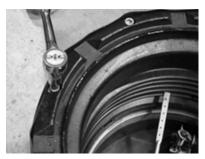
Step 8: Use a ratchet with a 9/16" socket to remove and discard all eight 3/8" stainless steel bolts located along the top of the rim of the A1004EVR spill containment.
