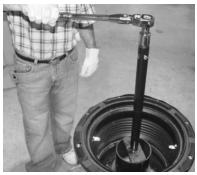
Step 6: Use the EMCO Adapter Wrench p/n A0081-001 to loosen and remove the 494096 riser seal.
