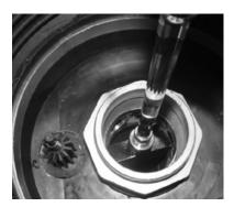
Step 5: Use the EMCO Riser Seal Wrench p/n A0081-001L to loosen and remove the center insert located inside the 494096 riser seal.
