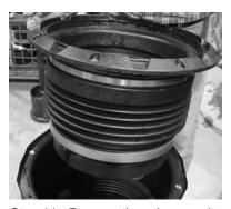
Step 11: Remove the primary unit from inside the A1004EVR spill containment by pulling upwards. Once the primary unit is completely out, please discard.
