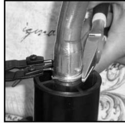
17. Use the snap ring and needle nose pliers to install the new snap ring into the machined groove located on the spout. Slide the snap ring downward until seated properly.
