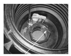
**Step 5:** Test fit the new stainless steel liner to ensure that it sits completely flat on the top of the rim surface. If the riser pipe is not visually straight up and down, it is possible that the liner will not seat properly. Rotate the liner as required to ensure proper alignment with the riser. Remove the liner.
