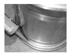
**Step 6:** Thoroughly clean the existing rim surface with a wire brush, then with a solvent such as lacquer thinner to ensure there is no oily residue on the rim. A bead of urethane sealant, placed on the underside cavity of the stainless steel liner, may be used to prevent groundwater from entering the existing containment.
