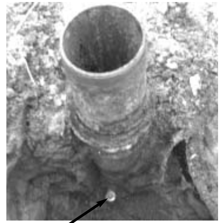
Hose to riser pipe connection plugged (using a 3/8" pipe plug).
