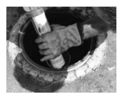
**Step 10:** Thoroughly clean the existing rim surface with a wire brush, then with a solvent such as lacquer thinner to ensure there is no oily residue on the rim. A bead of urethane sealant, placed on the underside cavity of the new bucket, may be used to prevent groundwater from entering the existing containment.
