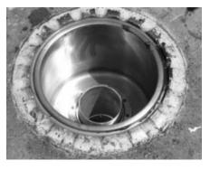
**<u>Step 11:</u>** Install the new stainless steel bucket over the nipple, pushing it down completely to ensure that it seats fully on the existing rim.
