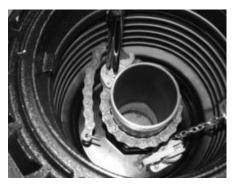
**<u>Step 7</u>:** Remove existing pipe nipple. Clean with a wire brush. Use a chain wrench to re-install the nipple or a new nipple if required. Avoid scarring the seal surface. (If seal surface is damaged, the unit will not pass pressure decay test.) Use pipe sealant on the lower threads. Repeat steps 2 and 3 to insure proper nipple selection.
