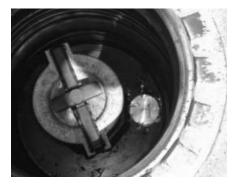
**Step 8:** Using a 1/2" socket, remove the drain, if existing. Carefully inspect the drain cavity to ensure there is no damage that could cause the bucket to fail testing requirements. Plug the drain cavity using Emco A1005-505DP or A1005-505DPE (w/epoxy) Drain Plug Kit, following instructions included with kit. If using A1005-505DPE, insert drain plug (included in kit) into drain channel to prevent flow of epoxy.
