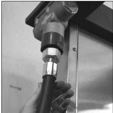
3. Install the standard whip hose into the adapter nut.
