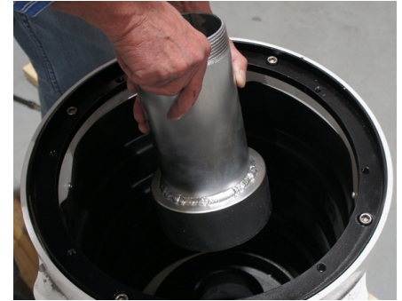
Step 9: Install the riser extension onto base flange. Tighten securely.
