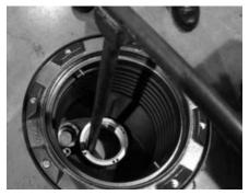
**Step 3:** Remove primary unit using the A0081-001H Wrench by inserting the wrench into the drain channel. Discard primary unit.
