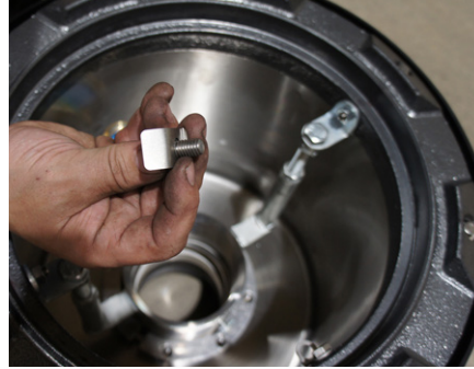
Step 8: Use the eighth bolt to install the grounding clip. The grounding clip must touch the riser pipe. Hand tighten all eight bolts.
