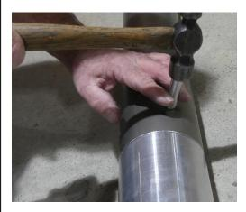
Step 4: using only the factory supplied pop rivets, apply a generous amount of Seal-All Sealant around the base of each pop rivet before installing into each of the four holes. Using the pop rivet gun, permanently fasten the A1100 riser collar to the top of the drop tube.
