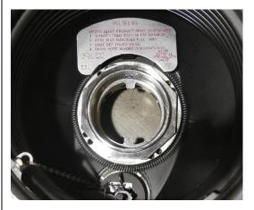
**Step 3:** reinstall the fill adapter onto the riser and tighten. Do not use pipe dope on the threads as the adapter seals on a gasket. Torque to 60-75 ft. lbs.
