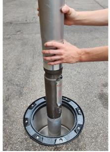
**Step 1:** Remove the cap and adapter. Raise the valve assembly out of the tank as shown. Use an assistant to hold the valve in position during the testing.
